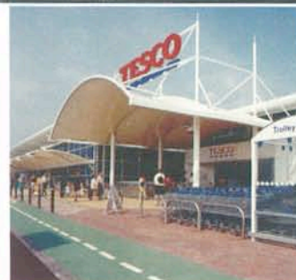
PAGE 30 Energy savings at Tesco Express
